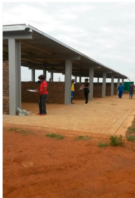
Figure 7. Shade provided on a landfill. Source: Authors.
