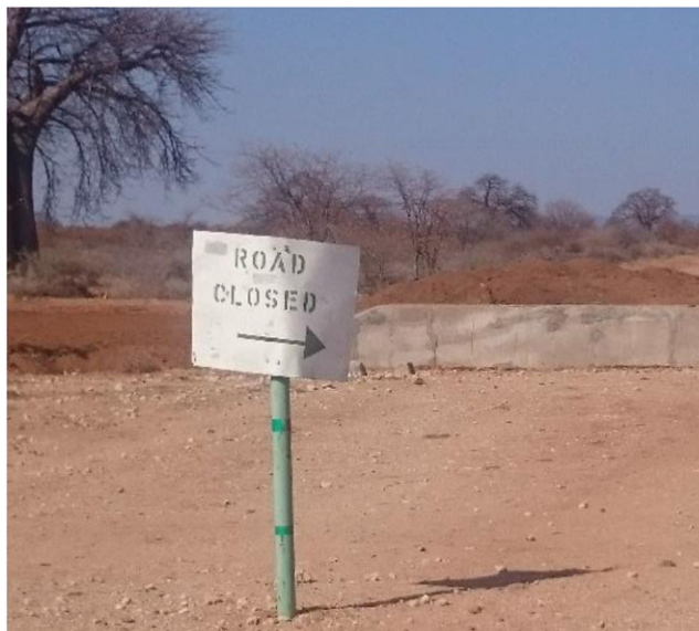
FIGURE 3 Road under maintenance in the study area
