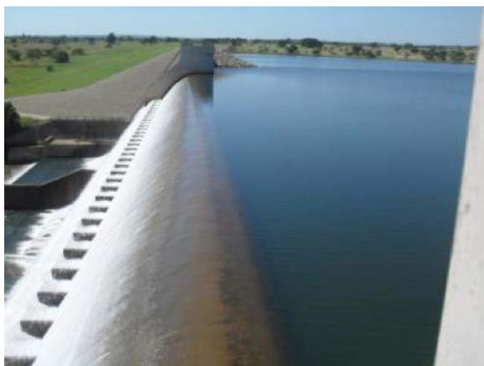
Figure 45 Driekoppies Dam wall
