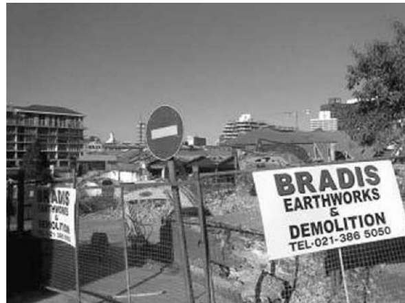
Fig. 8 Demolition site, corner of Napier and Jarvis Streets (June 2007)
