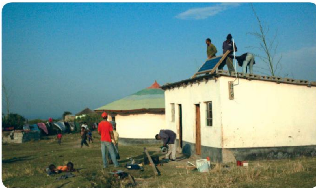
Installing a network node in Mankosi.
