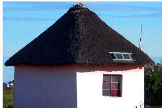
Figure 1: Solar panel and mesh router unit
