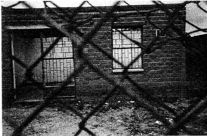
Figure 1: A derelict building known as a suiker huisie (sugar house)
